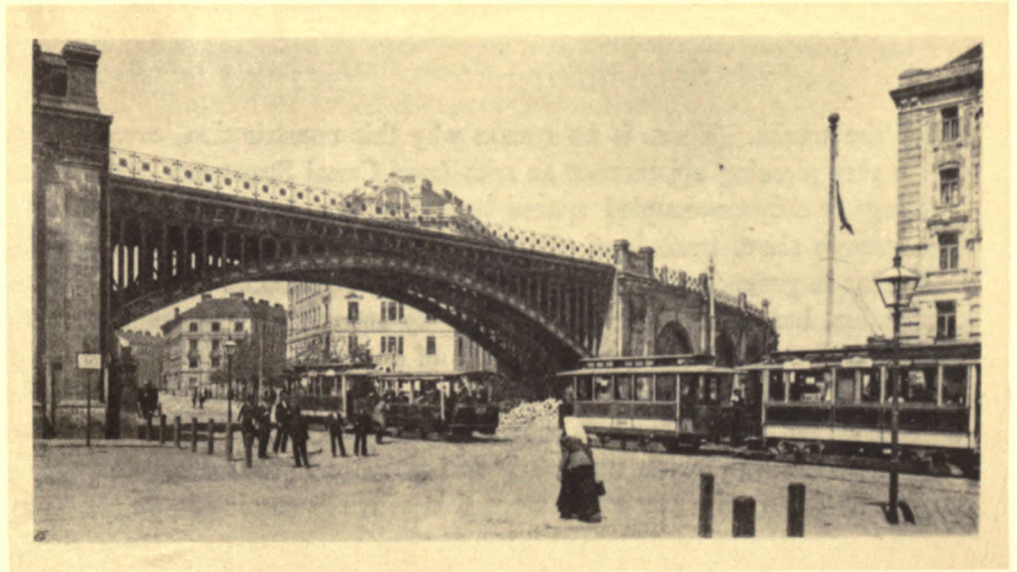
LXXVII. VIENNA. A RAILWAY VIADUCT PASSING OVER AN IMPORTANT STREET.
