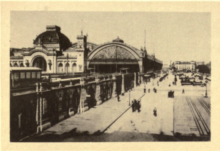
LXXVI. DRESDEN. VIADUCT AND RAILWAY STATION (HAUPT BAHN-HOF) PASSING ABOVE THE NORMAL STREET LEVEL, ILLUSTRATING THE TYPE PROPOSED IN THE OVERHEAD SCHEME FOR RAILWAY STATIONS WEST OF THE RIVER.
