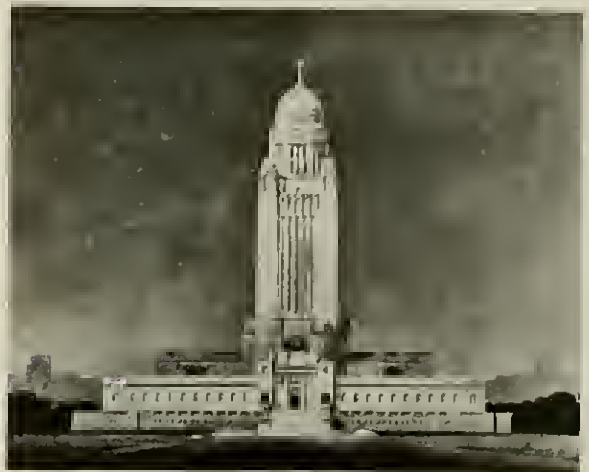
FIG. 602—LINCOLN. NEBRASKA CAPITOL COMPETITION The winning design, submitted by B. G. Goodhue. The site consists of four city blocks at the intersection of two important avenues. Mr. Goodhue's plan is a cross within a square, 360 feet over all. The design submitted by McKim, Mead, and White and by H. Van Buren Magonigle fit pretty nearly the entire site, which is 720 feet square. All of these designs show a remarkable independence of state capitol traditions. The official and popular approval with which that freedom has been received is perhaps due to the educational effect of the Cull-fornia fairs, which demonstrated the beauty of enclosed courts and the superiority of a spreading "system" of buildings over a single isolated monument. (Figs. 600-603 from the Architectural Review, 1920.)
