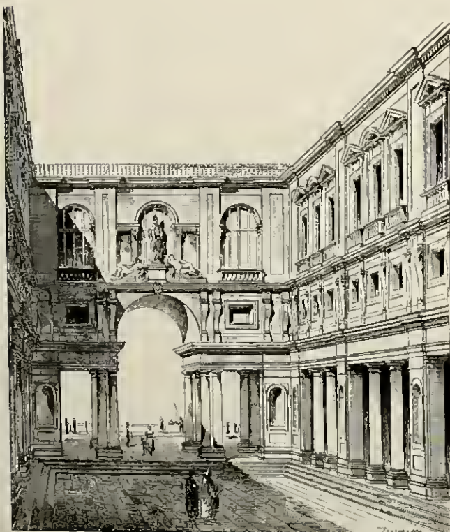
FIG. 21—PORTICO DEGLI EFFIZI, DESIGNED BY GIORGIO VASARI, 1560.
