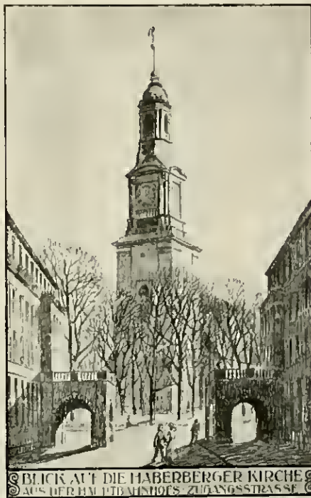
FIG. 694—KÖNIGSBURG. VIEW OF CHURCH FROM THE STATION SQUARE Designed by Förster. (From Stuedtelau 1916.)
