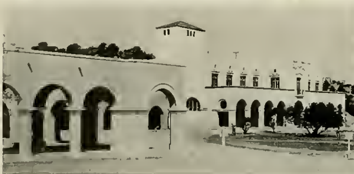
FIG. 483—TYRONE, NEW MEXICO. STORE BUILDING TO THE RIGHT, OUT-DOOR WAITING ROOM TO THE LEFT
