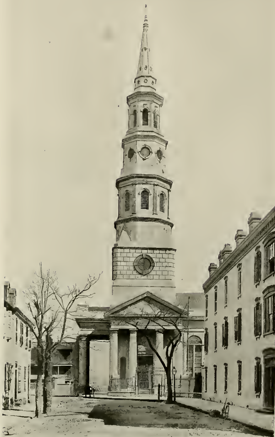
FIG. 719—CHARLESTON, S. C. ST. PHILIP'S CHURCH
