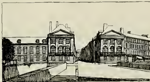
FIG. 705—ORLEANS. BRIDGE OVER THE LOIRE WITH DESIGNED ENTRANCE TO RUE ROYALE (From a drawing by Franz Herding.)
