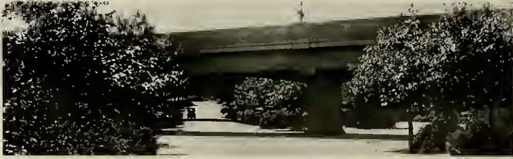
FIG. 841—BOSTON. ELEVATED RAILWAY CROSSING THE ARBORWAY AT FOREST HILLS
