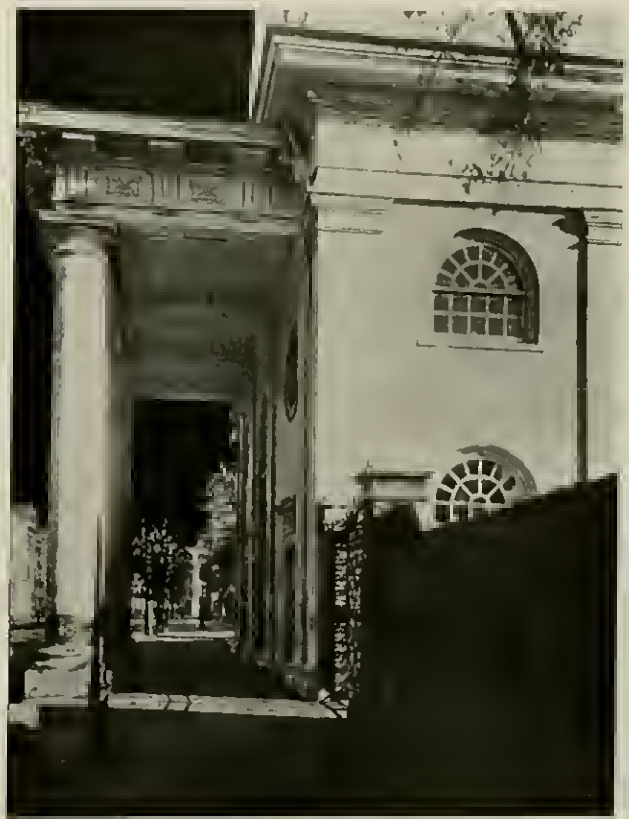
FIG. 714—CHARLESTON, S. C. ST. MICHAEL'S CHURCH The porch is brought over the sidewalk; see plan Fig. 715 and view Fig. 718. (From Ware's "Georgian Period.")
