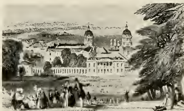
FIG. 6—THE GREENWICH HOSPITAL SEEN FROM THE HILLS An engraving dating from about 1840. In the foreground Lord Jotter's Queen's House and the colonnades tying it to the rest of the composition.
