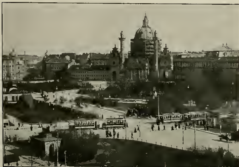
FIG. 295—VIENNA, ST. CHARLES CHURCH AFTER THE COVERING OF THE WIEN RIVER
