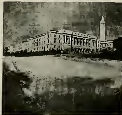
FIG. 508—VICINITY OF CAMPANILE
