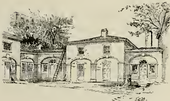
Yard and Stabling to the above
