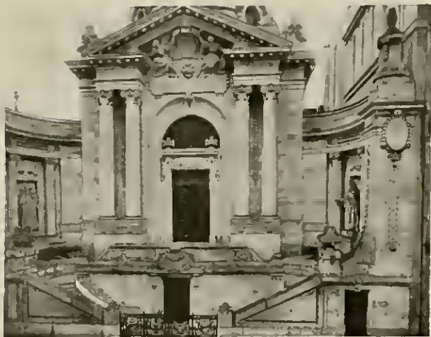
FIG. 720—PARIS. CHAPEL IN RUE JEAN GOUJON Designed by M. Gilbert. (From the Architectural Review, 1902.)
