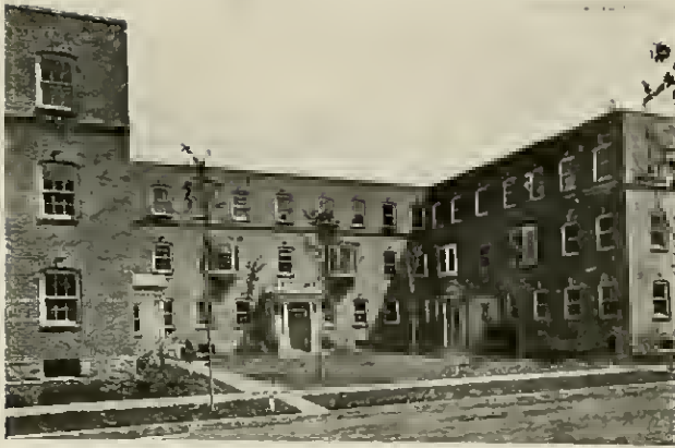
FIG. 1147—BRIDGEPORT. BLACK ROCK DEVELOPMENT Designed by B. Clipston Sturgis. See plan, Fig. 1148.
