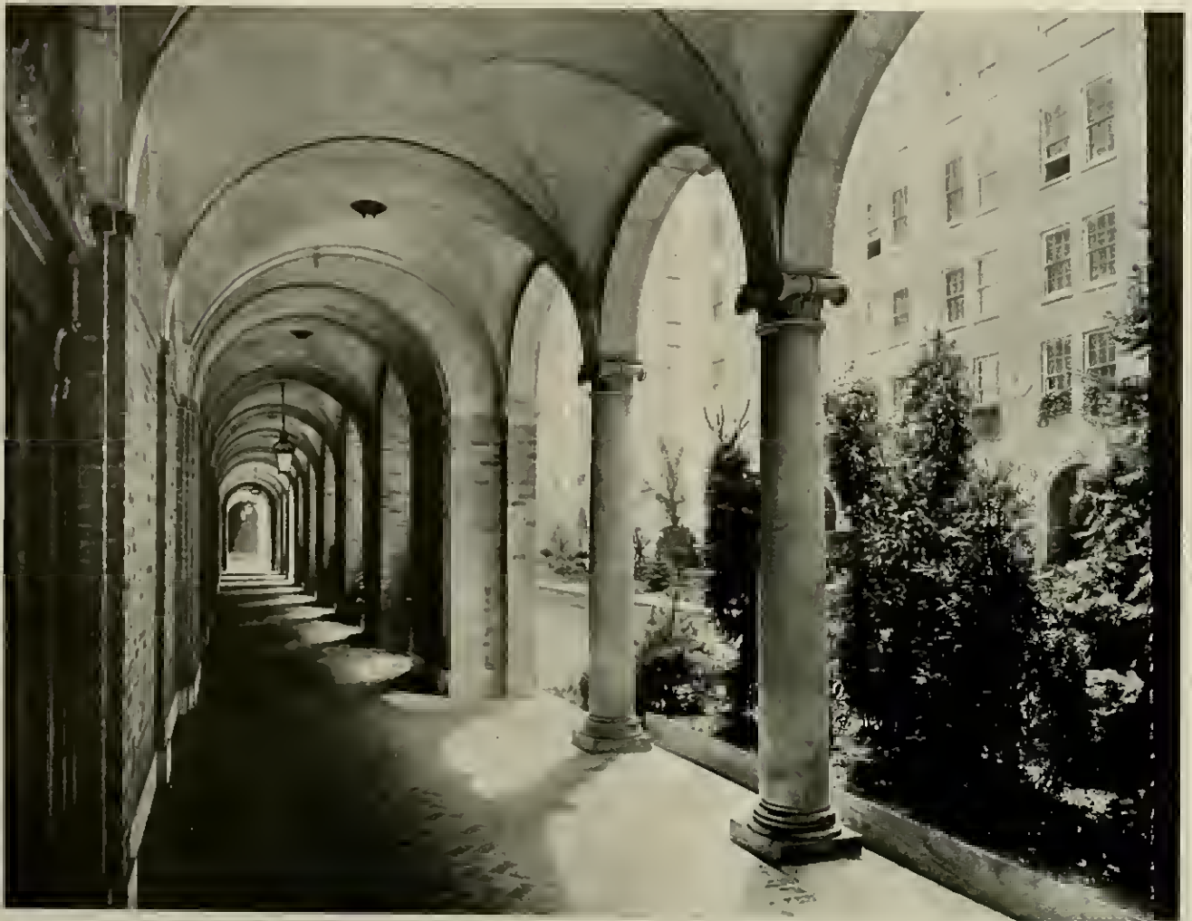
FIG. 832—NEW YORK. COURTYARD OF APARTMENT HOUSES ON PARK AVENUE Designed by Warren and Wetmore. See Figs. 833, 834.
