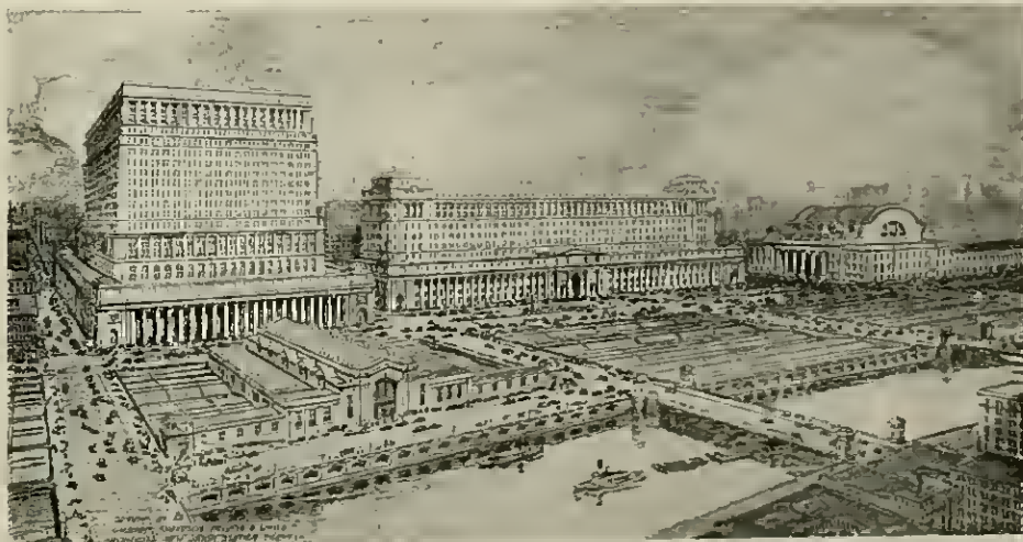
FIG. 806—CHICAGO. NEW UNION STATION
