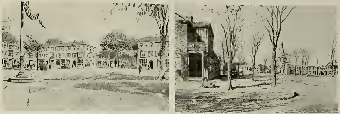
FIGS. 1138, 1139—YORKSHIRE VILLAGE, ALBERMARLE SQUARE AND NORTH COMMON Houses for shipping workers near Camden, designed by Eleonora D. Mitchell. (Figs. 1138-43 from the Architectural Forum, 1918.)
