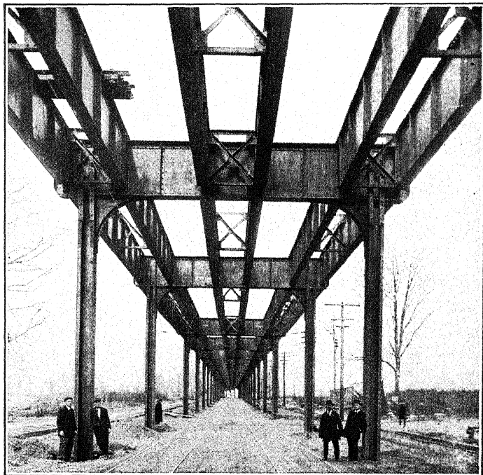
ELEVATED RAILROAD, STEEL STRUCTURE
